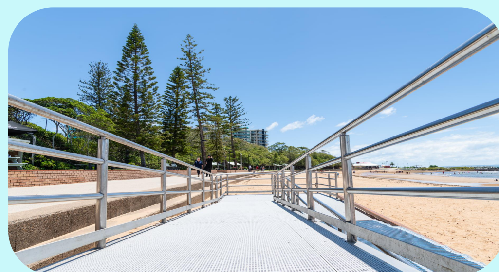
DDA compliant ramps with handrails
